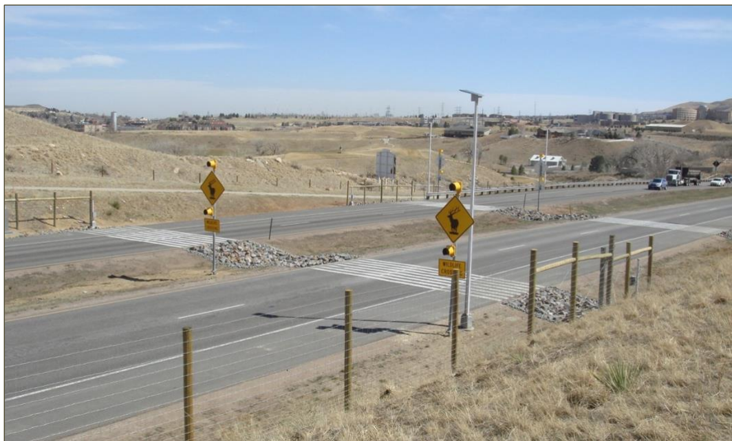
Figure 3. At-grade crosswalk system on US 6. Photo credit: CDOT
